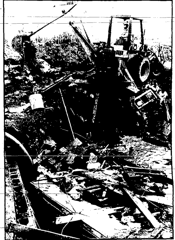
Spring cleaning TWO BUILDINGS located at the corner of 5th Street and Dearborn in Wayne were destroyed — one by fire and another torn down — to make room for a new 10,000 square foot True Value business. Above, a backhoe operator removes debris from the basement of one of the razed buildings. Photography: Chuck Hackenmiller
